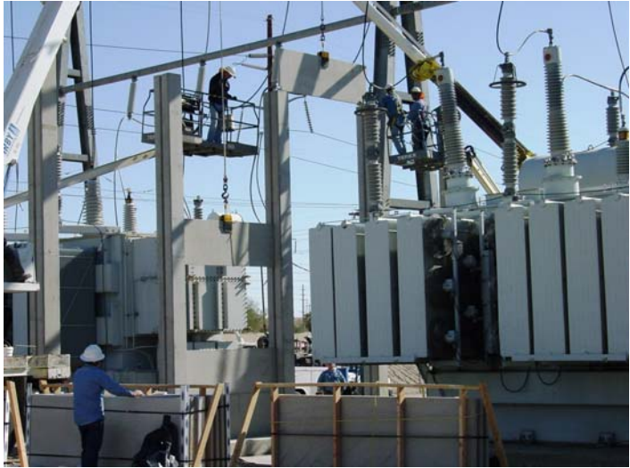
Step Two - Slide in the panels and ...
