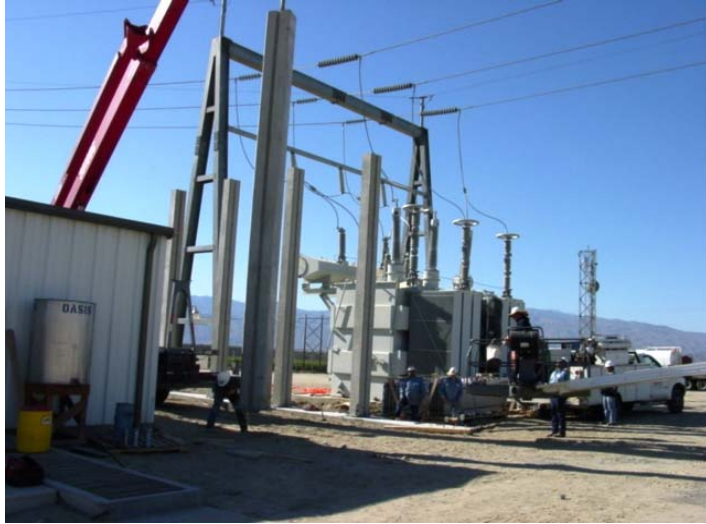
Step One - Position, align, and secure the columns.
